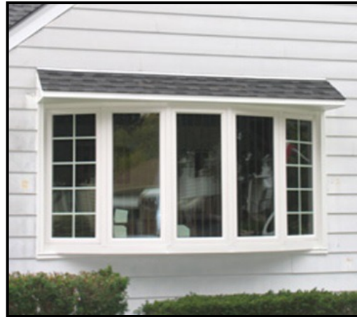
Typical "Box or Shed Style Roof, built on jobsite
